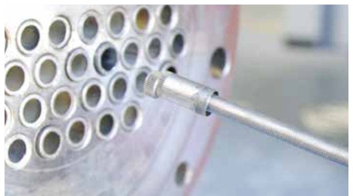
Thread a rod with a tube over top into the plug. Secure with washer & nut.
